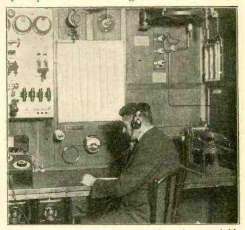
Fig. 4. Ship radio-telephone station designed on the new principle described herewith.
