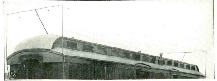
Exterior of car showing antenna equipment devised by Earl Hull, of the Oklahoma Radio Shop. It comprised four 4-wire cage antennas.
