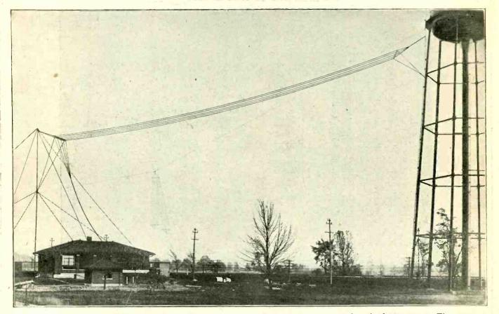
The Ford radio station, WWI, at Dearborn, Michigan. This station operates on a wave length of 500 meters. The antennae are a large inverted L and two smaller aerials. This makes long-wave reception possible with the large aerial. With the smaller ones, interference from neighboring stations can be practically eliminated.
