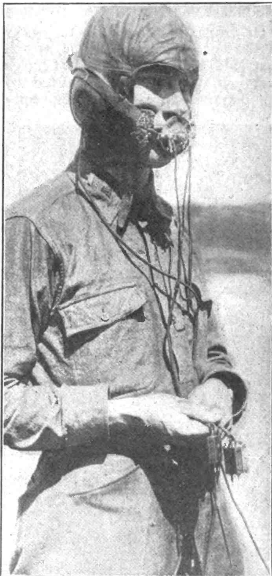
The above photograph illustrates a type of radiophone head gear, consisting of a microphone and a set of ear pieces, which fit snugly over the head. This is a marked improvement in radio for operators who work aboard airplanes. It is possible for the operator to manipulate the controls, dials, direction finder, and key without holding a microphone, which had to be done prior to the use of this device. The microphone is so adjusted before the speaker's mouth that he can use it without bending his head. Close inspection shows that it is not far from the lips of the operator. Voice tests have indicated that indistinct transmission of speech is produced when the operator wears the transmitter too far from his lips.
