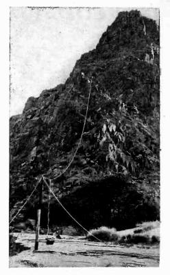
Antenna installed in Grand Canyon of Colorado River for receiving radio messages for the Geological Survey, U. S. Department of Interior.
