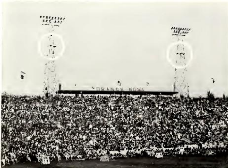
Famed Florida Orange Bowl gets its sound and light from the same supporting towers. Bob Lehfeldt of Flagler Radio Co., Miami, installed twenty Atlas Sound Corp. 8-inch cone size trumpets to cover the field.
