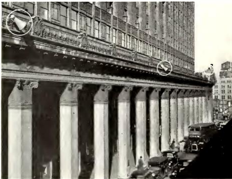
Unique car calling system recently added to the Chicago Civic Opera Building halves time required to empty the 3600-seat house. The doorman can quickly call any car, by its identifying number, from a nearby parking lot as it is required. One 60 and two 25-watt speakers are used in the sound system installed by the RCA Victor Distributing Corp. under the direction of B. J. Sullivan.
