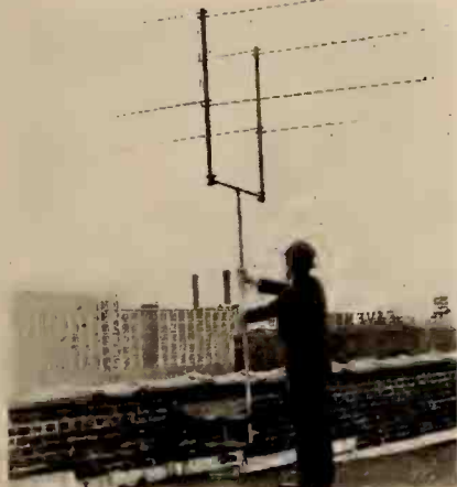
Double di-pole antenna of the RCA Mfg. Co., reduces "ghost" images.
