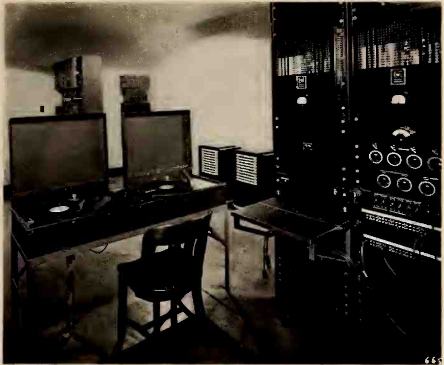
Control position of the centralized sound system supplying the Music Hall in Kansas City. Switching and mixing panels shown on the right and transcription tables on the left. Radio tuner also mounted in rack to the right.
