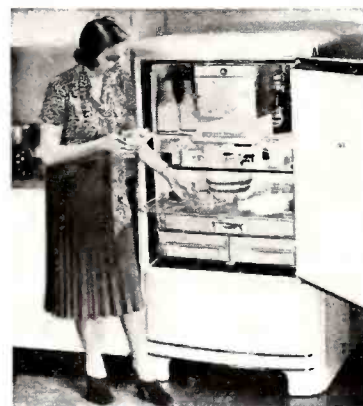
Frigidaire's Cold Wall is divided into 2 sections by a glass shelf.
