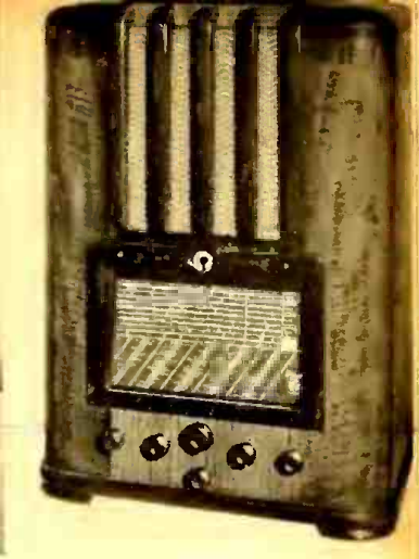
Pilot model TG528 12 tubes tuning to ultra-short-wave.
