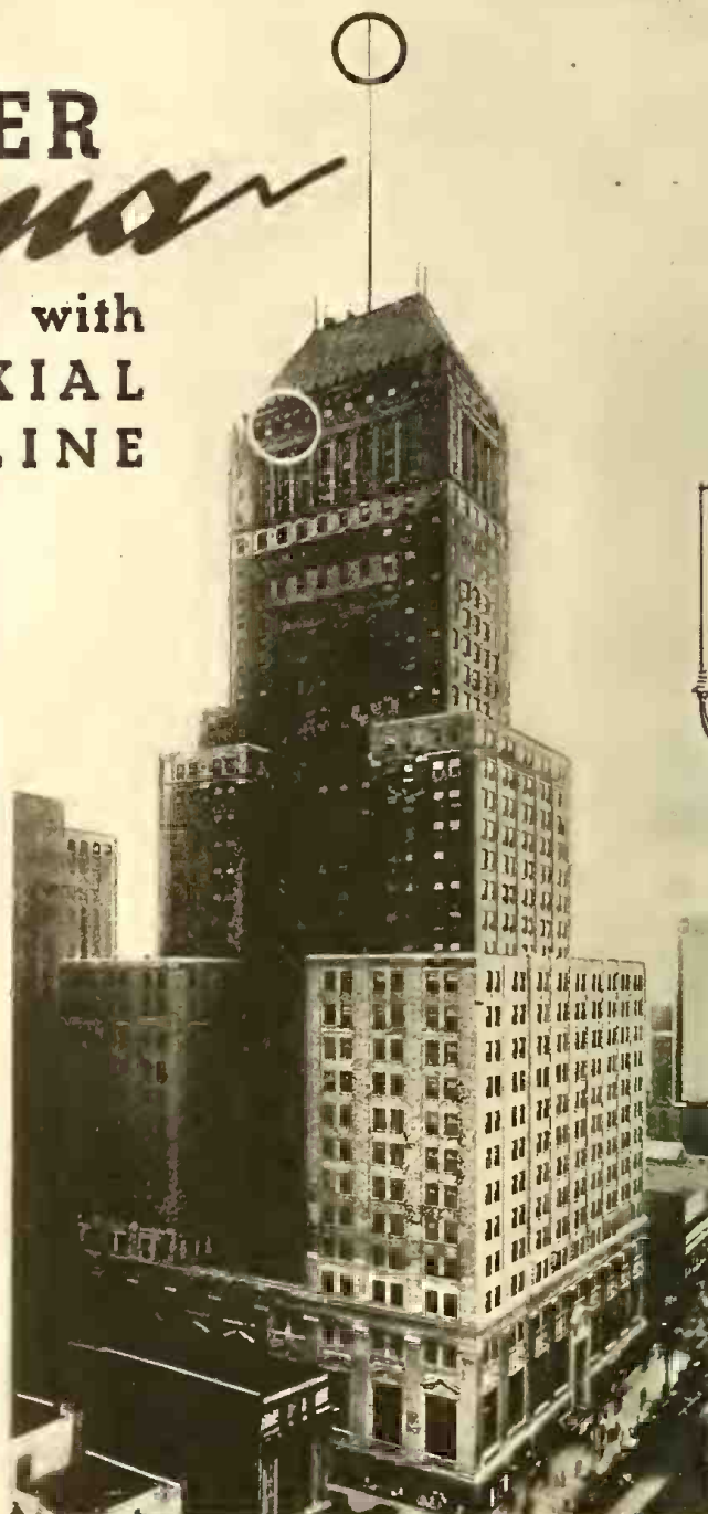
National Newark and Essex Bank Building. Showing location of transmitter and antenna connected by ISOLANTITE COAXIAL TRANSMISSION LINE.
