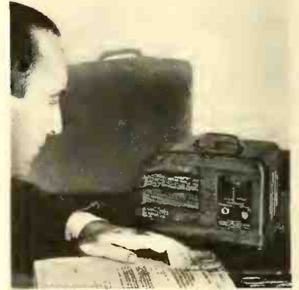
"Packaged communication." Plug this Carrier-Call into the nearest outlet, and talk to any other nearby outlet, over the electric-light wires!
