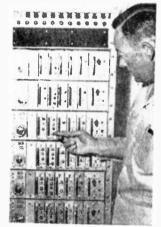
Banks of signal processors are part of automatic head-end operation. Devices amplify signals and sometimes switch channel frequencies.
