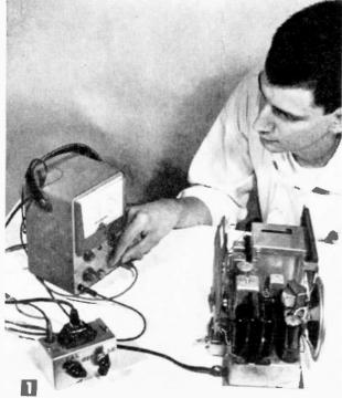
Author Lucos demonstrates haw "Mini-Amp" and sensitive VTVM can be used to abserve small changes in power consumed by radia. Unsteady reading indicates defective parts.
