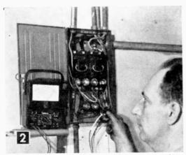
S&M consultant, Erving Edell checked out this method of reading power consumed in home circuits. It was easy to trace circuits, in any part of the building. The VOM is far more sensitive than the usual electrician's instrument and even a 25 watt test lamp added to an existing amperage on the dial was clearly seen on the meter's calibrated scale.
