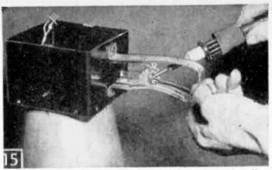
Soldering connections to switch terminals in handle of megaphone-see Fig. 5.
