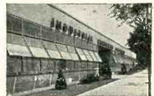
Modern plant built by Industrial Condenser Corp. for manufacture of capacitors only
