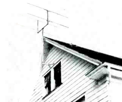
Fig. 6—Double di-pole and reflector
