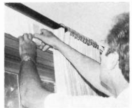
Fig. 6 Wireless transmitters can be installed in a matter of minutes—greatly reducing the installation time required. Although equipment costs will be greater when using wireless equipment, the savings in labor will more than make up for the higher costs.
