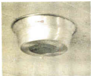
In many parts of our second building there are no false ceilings, thus requiring the use of dish-pan-type speaker enclosures.
