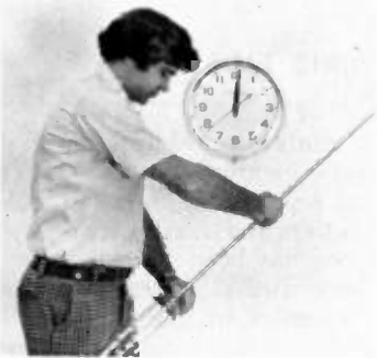
Tighten collar coupler, securing top radiator
