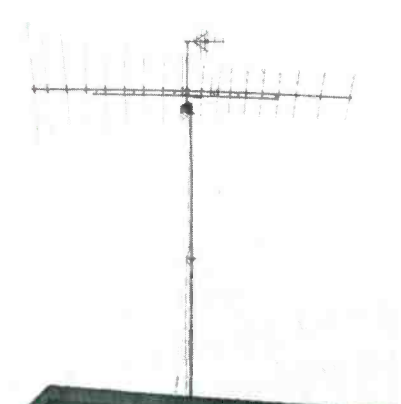
A typical Action Sales & Service home antenna installation.
