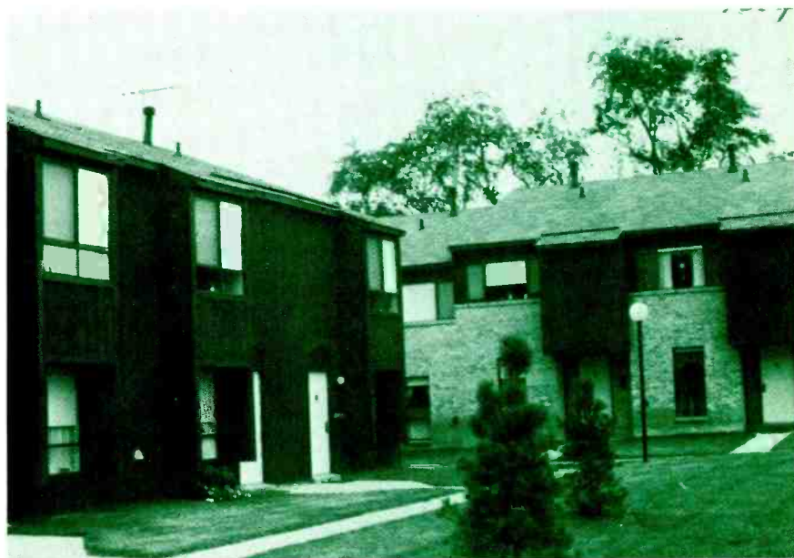
Part of the 200 - unit Dreshertown condominium, Wellener's first MATV job. Although his profit on this job was only 10 percent, Wellener gained valuable design and pricing experience, and the system works so well that Wellener uses it to show prospective customers the quality and performance he is capable of delivering.
