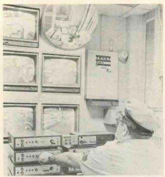
Communications center at Baker/Beech-Nut Corp. plant in Canajoharie, N.Y. with security officer monitoring five Motorola CCTV cameras as they observe virtually all of plant area. Center also includes radio and paging dispatch facility.
