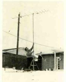
Rough orientation, once the test antenna is up, is the first step in determining the direction for best signal reception.
