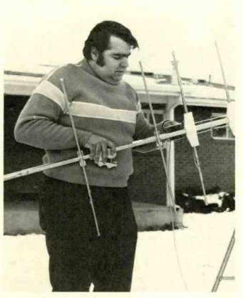
Joe Barno, Denver area MATV contractor, connects a down-lead to the test antenna in preparation for determining the available TV signal at an installation site.
