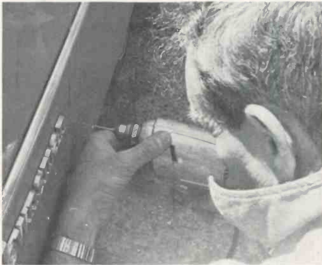
Fig. 13—Drilling antenna-mount holes.
