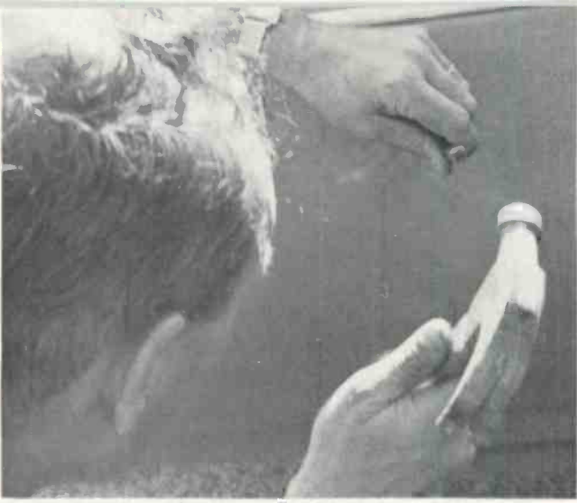
Fig. 12—Center punching antenna-mount holes for drilling.
