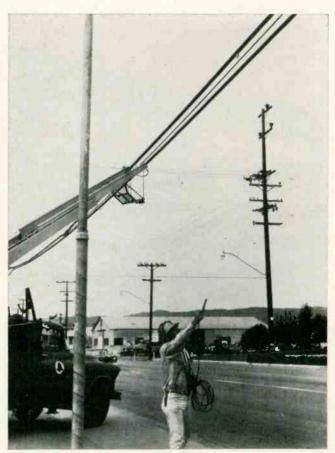
Maintenance man probes for leaks with a compact ultrasonic detector manufactured by Delcon Corp.
