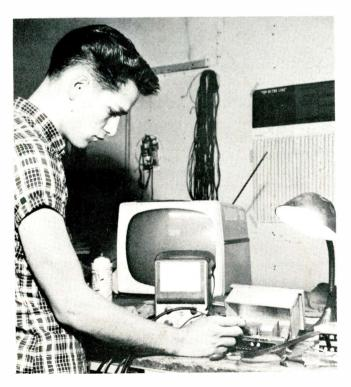
Checking out a topside antenna booster.
