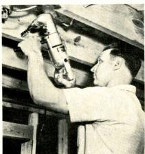
Sound system installers find this drill made by Black & Decker particularly valuable where cables must be run through joists.
