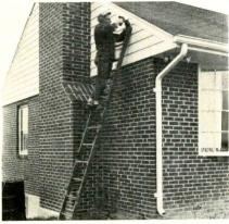
Battery-powered drill comes in handy for antenna installations.
