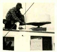
Technician installs radome on Raytheon radar antenna atop small cruiser.
