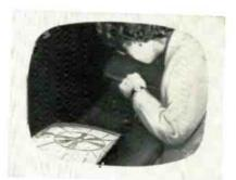
Screen inspection. Every completed Silverama is reinspected for screen quality and sharpness of focus at this special automatic testing station near the end of the production cycle. Each Silverama undergoes as many as 26 inspections before it is released for sale to your customers.
