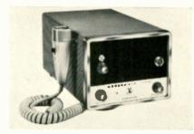
"Messenger," but includes a number of new features. The unit is designed for coverage of any 10 channels in the 23 channel band, has an illuminated channel indicator, and permits instant selection of any one channel by simply rotating the channel selector switch. The receiver section has been designed to offer increased sensitivity and high adjacent channel rejection. Transmitter circuitry has been designed for more than twice
