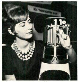
A thermoelectric generator is embraced by Maureen O'Donnell, while gazing at a nuvistor. Both devices were displayed at the annual IRE show in New York. The generator is under development by Atomics International for the Atomic Energy Commission. The device will use modules made from a new RCA thermoelectric alloy.
