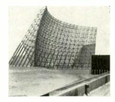
Fig. 3—One of the four giant long-range radar antennas, each 165 feet high and 400 feet long, used in BMEWS missile detection system located at Thule, Greenland.
