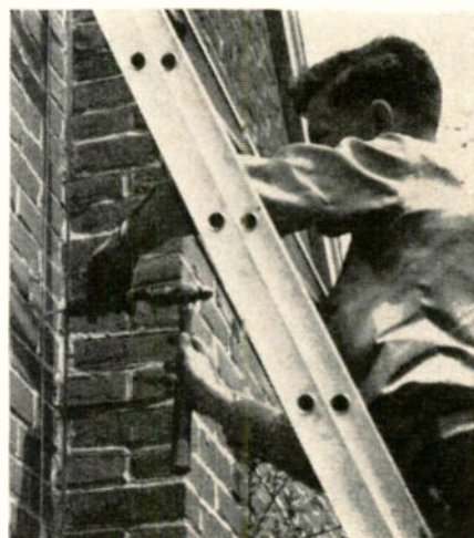
Fig. 6—Masonry bits are used to hammer holes in brick or mortar. A rotating action of the brace prevents tool wedge.
