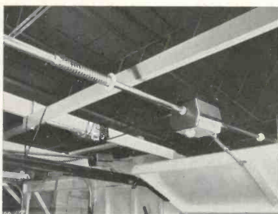
Perma-Power GDO installation in garage.
