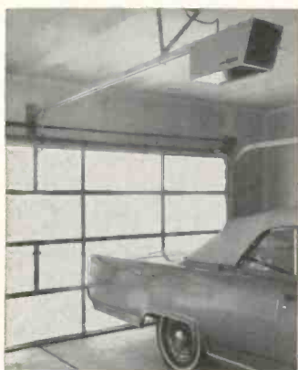
A Stanley-Berr model BA6 GDO mounted in garage.
