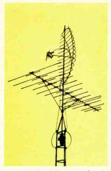
This cylindrical parabolic, mounted above the VHF antenna, gives very good results on channel 21 and 25 at 35 miles away.
