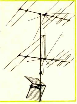
Fig. 1—UHF antennas mounted below VHF antennas make it difficult to get good reception.
