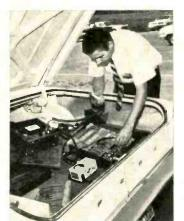
Field alignment is performed on mobile unit in police cruiser trunk. Touch-up tuning is frequently accomplished without removing unit.
