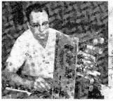
Advanced Engineering. Scott quality begins in the laboratory where the Advanced Development Team pioneered Wide-Band Design and "Time-Switching" multiplex circuitry. Chief Engineer Daniel Von Recklinghausen is shown here with the original model of the world's first commercial: FM Stereo signal generator, which is used by manufacturers throughout the world.
