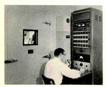
This Shure Brothers sound room is where the company is developing special-purpose mikes that can be used in noisy environments. For example, inside the  $6\times 6'$  insulated room, engineers can duplicate the room of a jet engine at 500 feet, unbearable to the human ear except for a few minutes.
