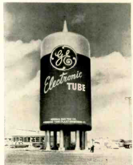
Built to the proportions of a 6BK7 (though 84,000,000 larger) this 200,000-gal. water tank at General Electric's new Owensboro, Ky., tube plant under construction is 80 ft.
