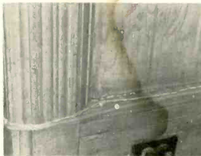
Fig. 7—More tacks to change line characteristics, as well as phone line to unbalance it.
