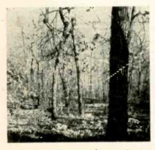
Fig. 1—Open-wire strung between trees on way down. Slack allows for tree movement.
