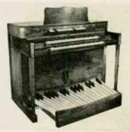
cept the keys and controls. Features the use of 130 printed circuits. Kits for the separate components, such as each of the 12 tone generators, or preamplifiers, stop filters, and so on, may be purchased separately to make budgeting easy. The Schober Organ Corp., 35 Dail St., New Hyde Park, New York.—TECHNICIAN (Ask for No. 6-66)
