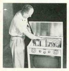
1955 line of Setchell Carlson receivers should make a big hit with TV techs. Chassis—all plugin units—is mounted under hinged IId. Units are Indivually removed for servicing. Tube replacements are made from standing position.
