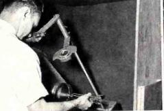
Examination with polarimeter permits careful control of strains for superior glass-to-metal sealing.
