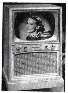
on new Power-Master chassis, with 24 tubes, including picture tube and 2 rectifiers, set will sell for \$379.95. Bendix TV and Radio, E. Joppa Rd., Baltimore 4, Md.—TELEVISION RETAILING.
