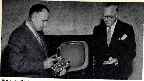
Part of Zenith's demonstration for the FCC of UHF television reception on Zenith receivers, was to show how simple it is to slip a UHF tuning strip into the turret tuner in every Zenith TV set. G. E. Gustafson, left, Zenith's vice-president in charge of engineering, holds one of the turret tuners. H. C. Bonfig, vice-president and director of sales, has one of the UHF
