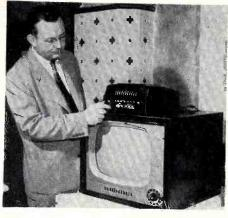
J. F. Walsh, sales manager of Westinghouse Electric Corp., looks over the firm's new UHF converter. It can be connected to all Westinghouse TV sets now in use, to enable them to receive all UHF channels.
