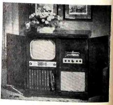
3-speed record changer, this model includes a 16-inch black-face rectangular tube TV set. Priced at \$565 complete, it is also available for \$329.50 in an Add-a-Vision model for later installation of the television chassis. Cabinet is dark mahogany, with two full-length doors and record storage space. Phonograph compartment is the lift lid type. Scott Radio Laboratories, Inc., 4541 Ravenswood, Chicago 40, Ill.—RADIO & TELEVISION RETAILING.
