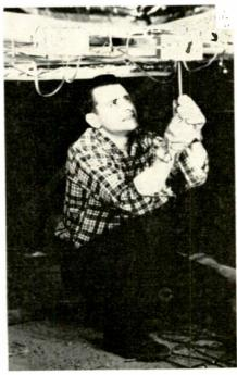
Basement installation of master antenna boosters. Maintenance is simplified by marking each twinlead with the apartment number.
