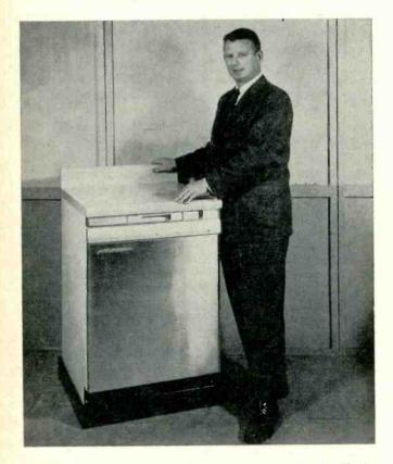
Ultrasonics, which has served science and industry so well, will now serve consumers directly in the form of this dishwasher made by Narda Ultrasonics Corp. Water is compressed and decompressed by 40 kc sound waves to cut the wash-dry cycle in half to 25 min. Initial price will exceed \$800, but should drop with volume production.
