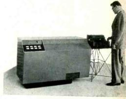
No larger than an office desk, this digital computer is designed to provide automatic control of industrial processes, data logging, and test facility operation.
