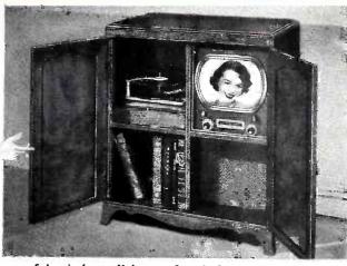
Sylvania 6-way Mahogany Console Combination # 128. 121/2" tube ... AM-FM radio ... 3-speed automatic record changer.
