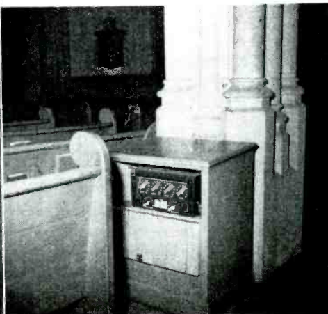
At left, the two altar mikes blend with their surroundings. Below, the specially-constructed case containing the amplifier and controls for the sound attendant matches the interior woodwork. At right, high above the pulpit, two speakers are entirely hidden behind miniature organ pipes. Because of strategic location, all the sound seems to come from the pulpit. Installation by McKee Electric.
