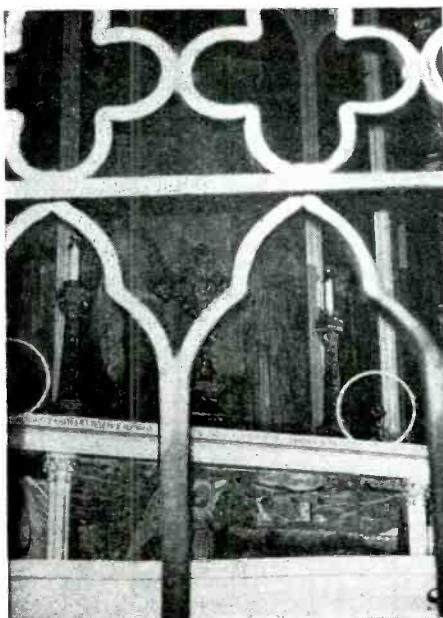
At left, the two altar mikes blend with their surroundings. Below, the specially-constructed case containing the amplifier and controls for the sound attendant matches the interior woodwork. At right, high above the pulpit, two speakers are entirely hidden behind miniature organ pipes. Because of strategic location, all the sound seems to come from the pulpit. Installation by McKee Electric.
